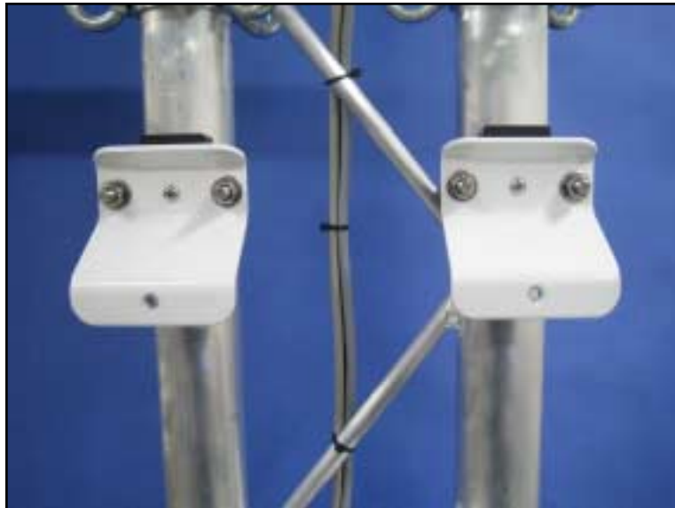
Figure 17: Connecting the cable bunch to the crossbars
